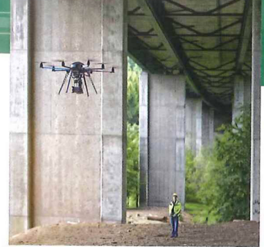
The high-tech mini-flyer scans entire buildings in just a few hours. Photo: Uwe Bellhäuser
